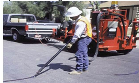
Figure 33. Filling cracks in initial stages of their formation [5].
