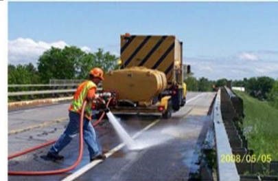
Figure 32. Pressure washing the drainage system [5].
